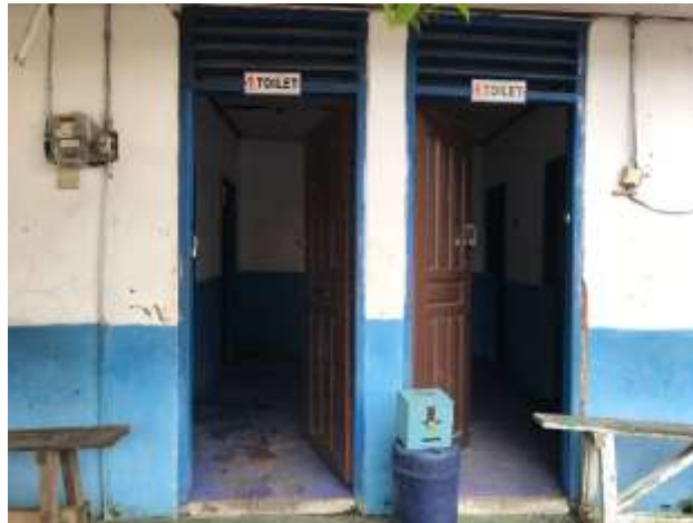
Gambar 5.29 Fasilitas Terminal Bus (Toilet)
