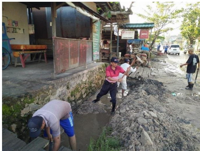
Figure 4. Cleaning Drainage Channels By the people in Lempake.
