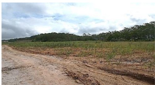
Figure 2 Land preparation at Ex-Pit IPDa-Komodo 2010 (5,11 Ha)
