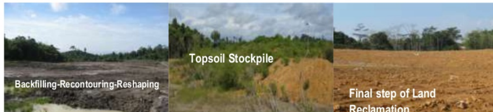
Photo-02. View of Study Area - Reclamation of Mined-out Lands of PT TCM, West Kutai, East Kalimantan
