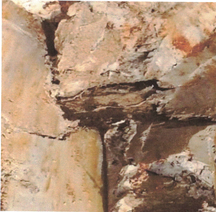
Figure4. Topsoil from marshland and crack formation (Crack Formation, < 2 years old)
