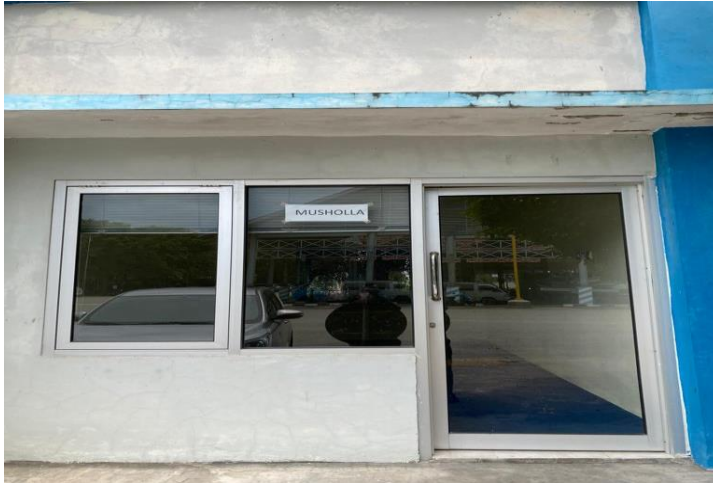
Fasilitas Mushola Terminal Bus Bontang
