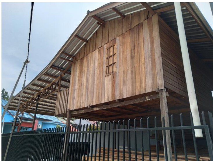
Figure 1. Wooden house in Samarinda, East Kalimantan. The wooden walls are nailed, and the support poles are screwed.
