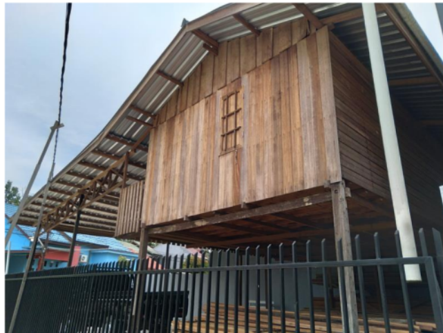
Figure 1. Wooden house in Samarinda, East Kalimantan. The wooden walls are nailed, and the support poles are screwed.
