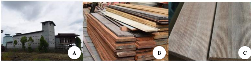
Figure 3. The structure of swiftlet house: A. The swiftlet houses; B & C wood materials to build swiftlet houses
