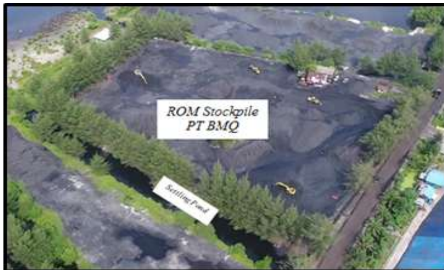
Gambar 2. Kondisi ROM Stockpile PT.BMQ
