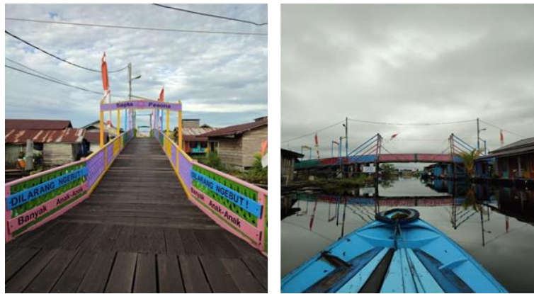
Gambar 5. Jembatan Desa Muara Enggelam Figure 5. Muara Enggelam Village Bridge
