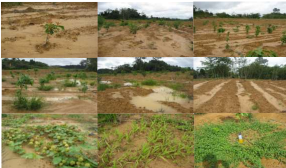
Photo-07. Initial Growth of Land Cover and Soil Erosion 3 Months After Revegetation Works
