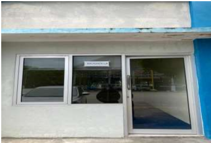
Fasilitas Mushola Terminal Bus Bontang
