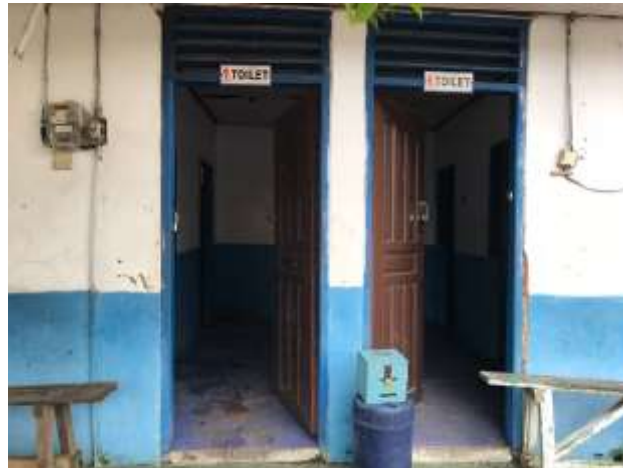
Gambar 5.29 Fasilitas Terminal Bus (Toilet)
