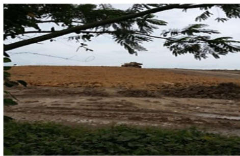
Figure 12. Massive impermeable layer and topsoiling processes of OB materials (topsoil processes).
