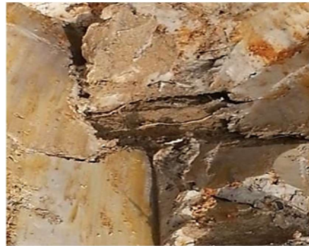
Figure 4. Topsoil from marshland and crack formation (crack formation, <2 years old).
