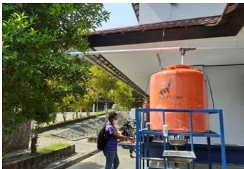
Gambar 2. Prasarana Metode Rainwater Harvesting
